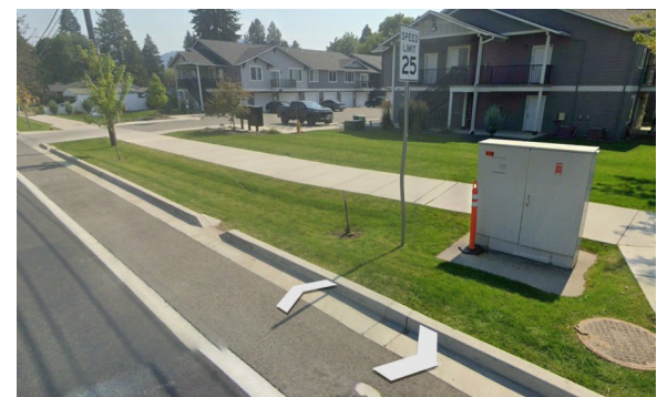
Frontage improvements constructed as a part of the Chubbs OPA
