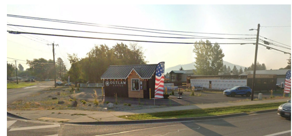
Marketplace at Miles OPA now has a building under construction and a new coffee stand.
